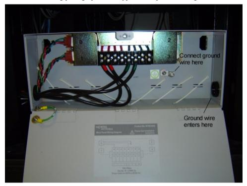
**Note:** The cables are marked with Red and Green tape. The cables with the Red tape connect to the Negative (-) Red side (on the left in the photograph), and the cables with the Green tape connect to the Positive (+) Green side (on the right in the photograph). The sides are identified on the power connections. The ground wire enters at the lower right and attaches to the ground lug.
